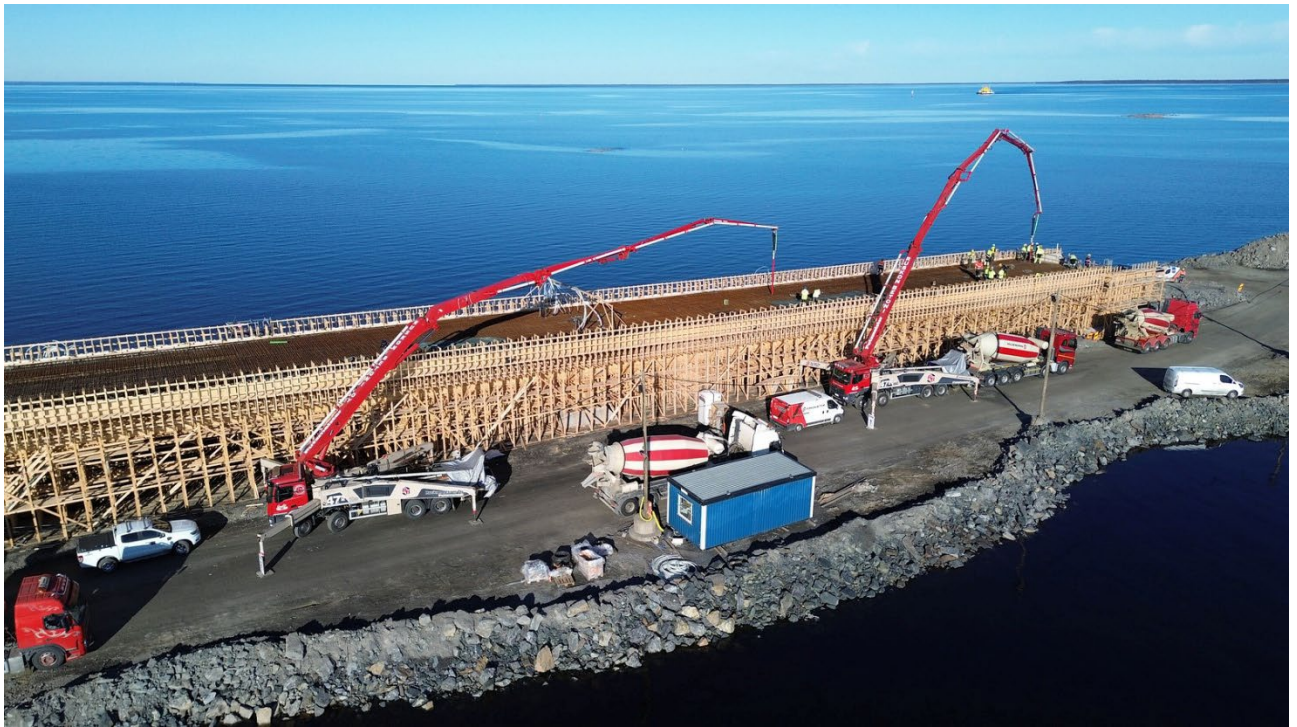
Two Putzmeister truck-mounted concrete pumps BSF 47-5 working on the Huikku Bridge
