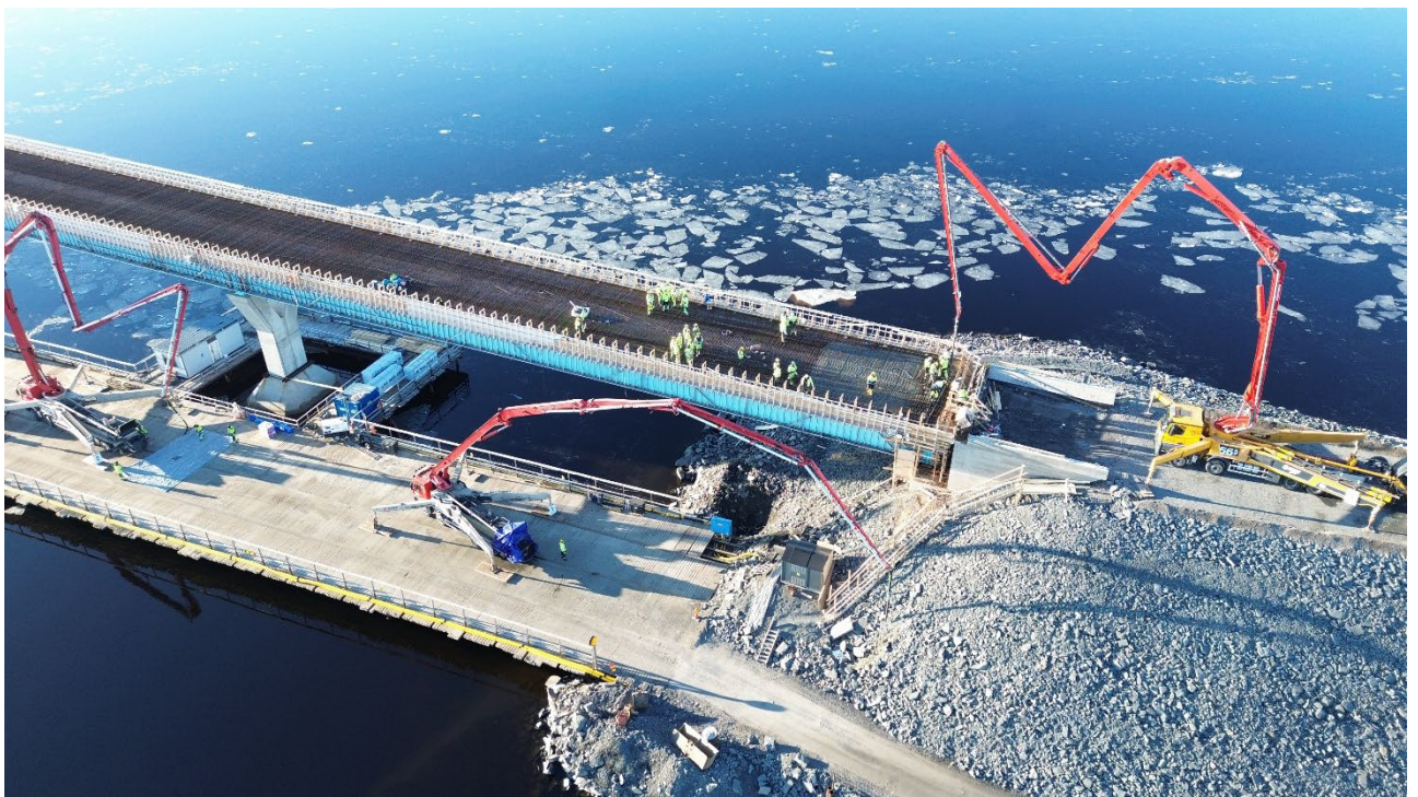
Putzmeister truck-mounted concrete pumps BSF 47-5 and BSF56-5 concreting the working on the Riutu Bridge
